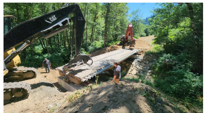
Railcar bridge installation on Tioga Creek tributary by TNT Construction & Excavation.
