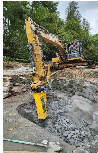
Left: Timber Roads, LLC widening jump hole at base of falls. Right: Fish tails at base of new channel dug into Tioga Falls.
