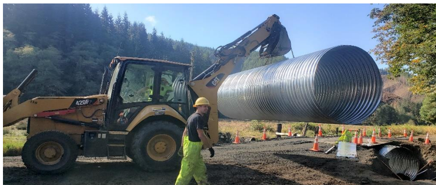
Stream crossing upgrade in the Palouse basin (24" pipe to 6' culvert).
