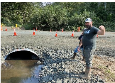
Newly replaced culvert feeding into Kentuck Creek.
